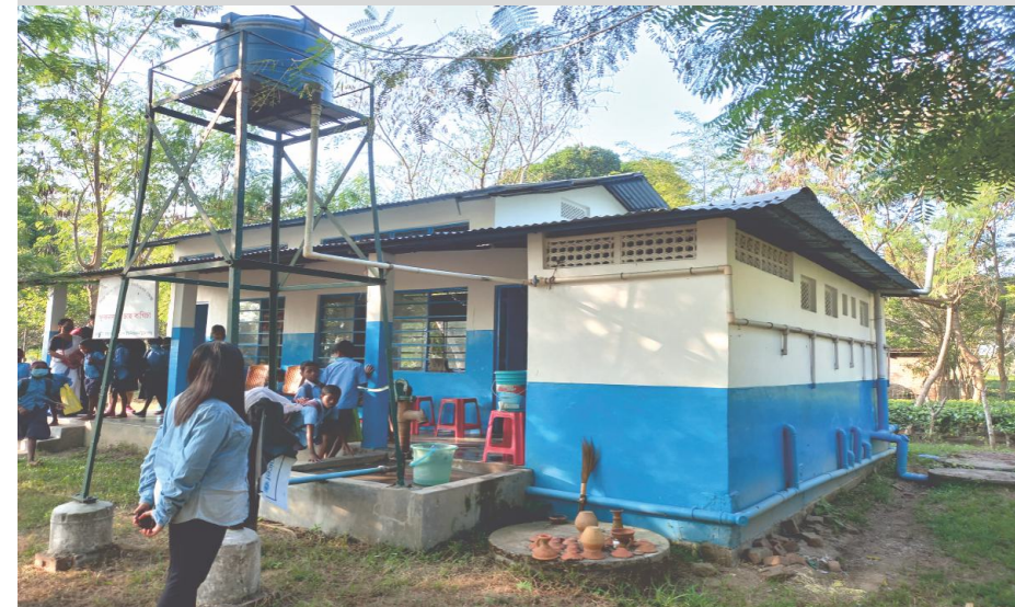
Photo 19 An ideal , functional School WASH facility, segregated for boys & girls
