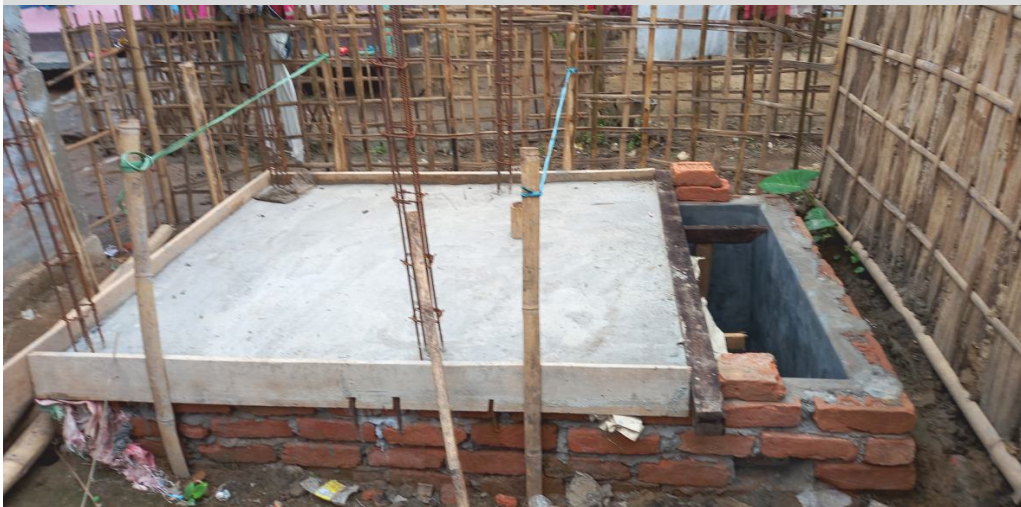
Photo 10 Septic Tank under construction - Owner driven effort
