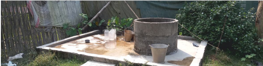
Photo 3 Tube Well - Hand pump with an Apron
