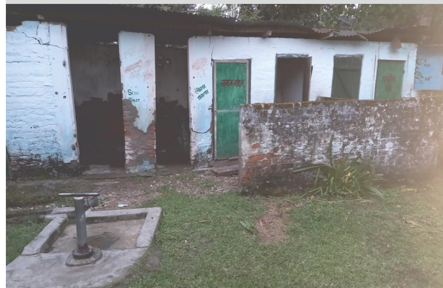
Photo 18 A hand pump used as drinking water source in the proximity of toilets in a TE school premises. Toilets were common, some lacked doors and were unclean
