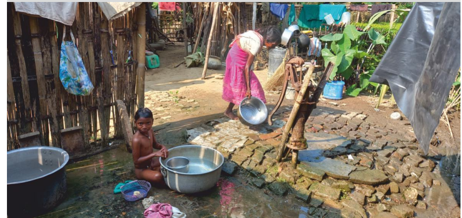
Photo 7 Hand pump in insanitary condition, potential risk of groundwater contamination
