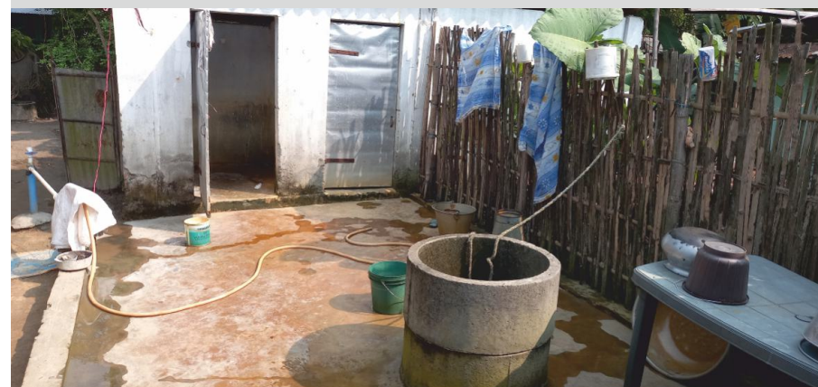
Photo 9 Inadequate distance between ground water source and toilet leach pits
